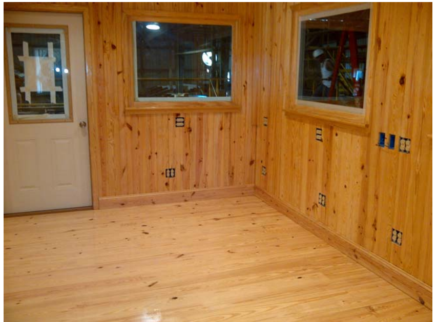
#2 V-Joint and flooring was used to construct our new computer room.
